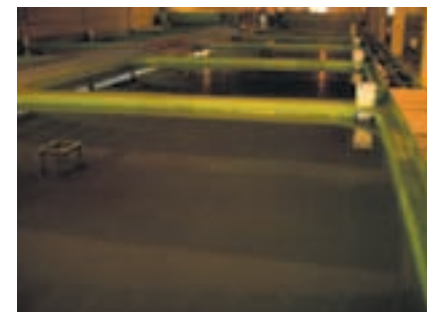
Tanks fully installed
